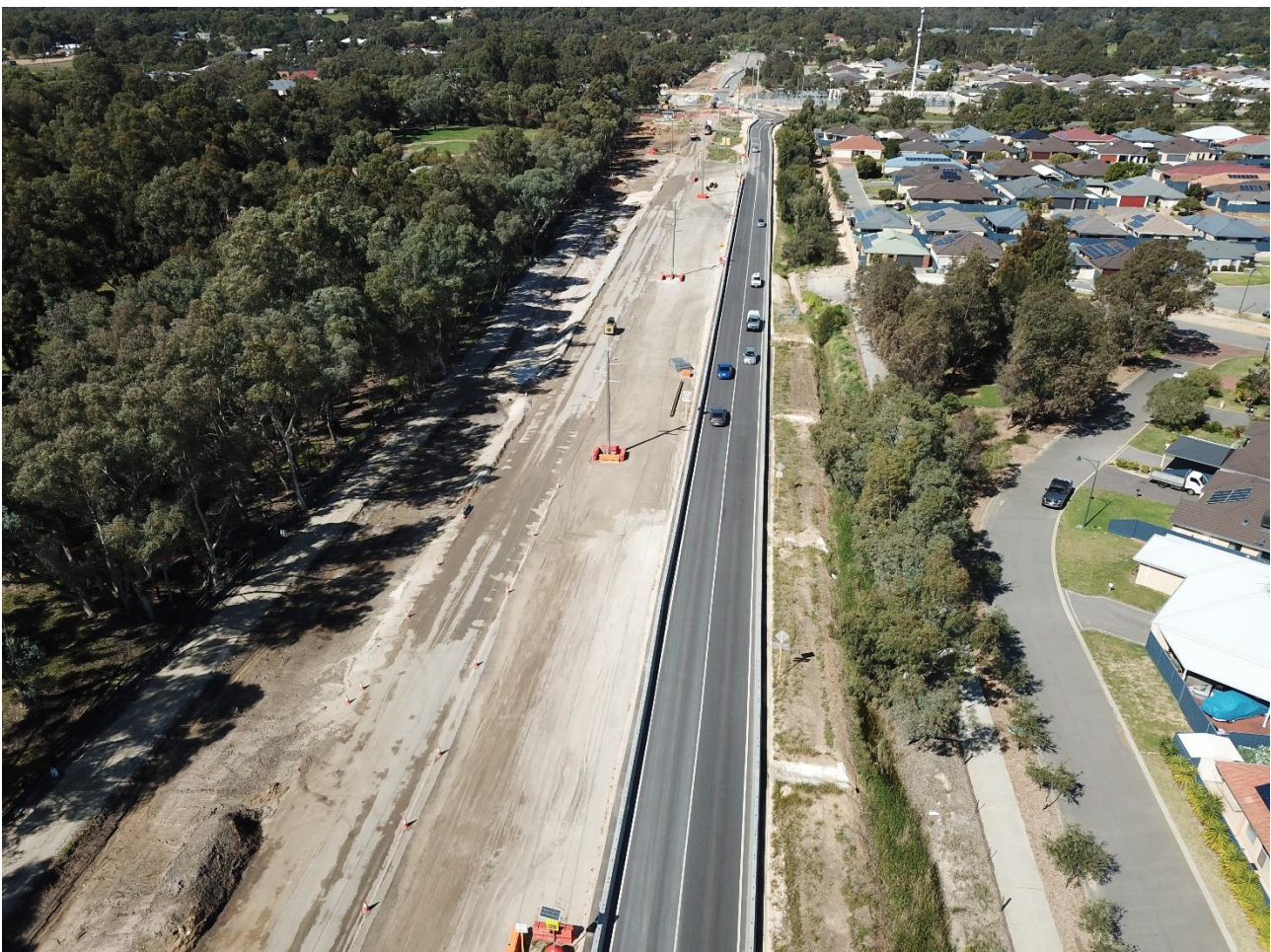
Figure 15 Existing Bridle Trail adjacent to Project works alongside property line
