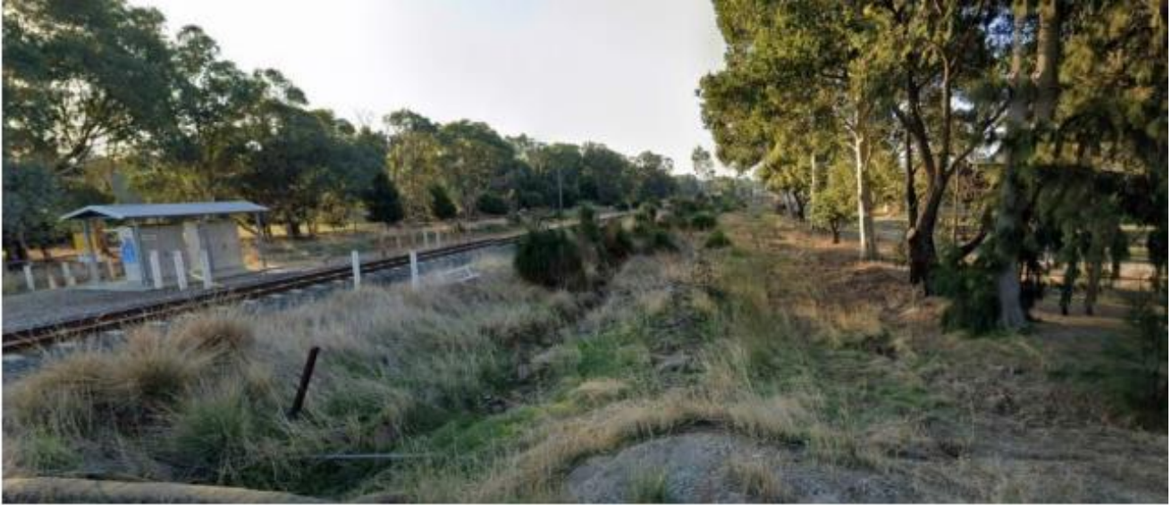
Figure 7 Rail Corridor facing north, showing completely degraded vegetation
